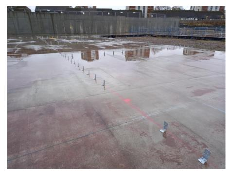
Brackets installed on lower ground floor slab ahead of cross laminated structure
